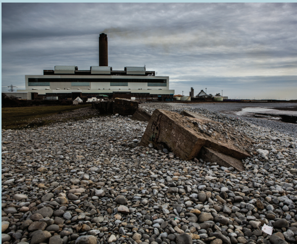
ABERTHAW POWER STATION, WALES, UK. © cliff hellis
